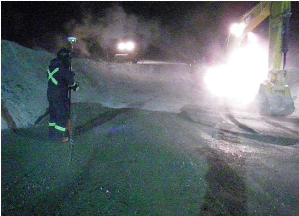
Photo 13: Survey picking up the edge of the FCM placed on nightshift.
