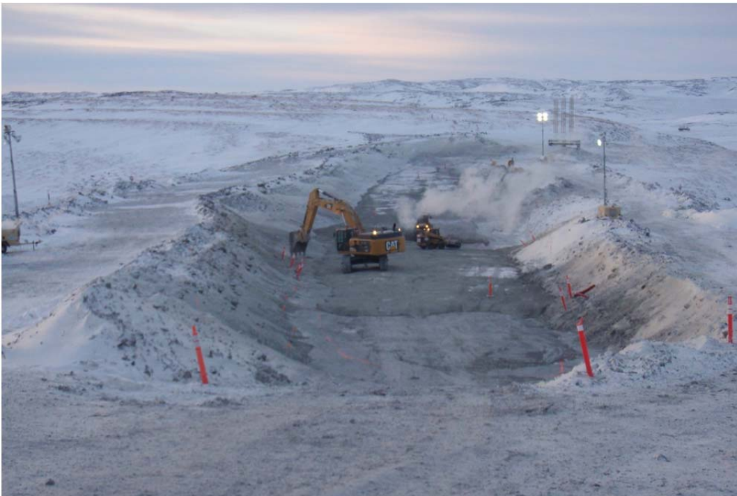
Photo 4: ~ WSW view of down the key trench. Note the skid steer and 345 excavator cleaning in preparation for placement in this photo.
