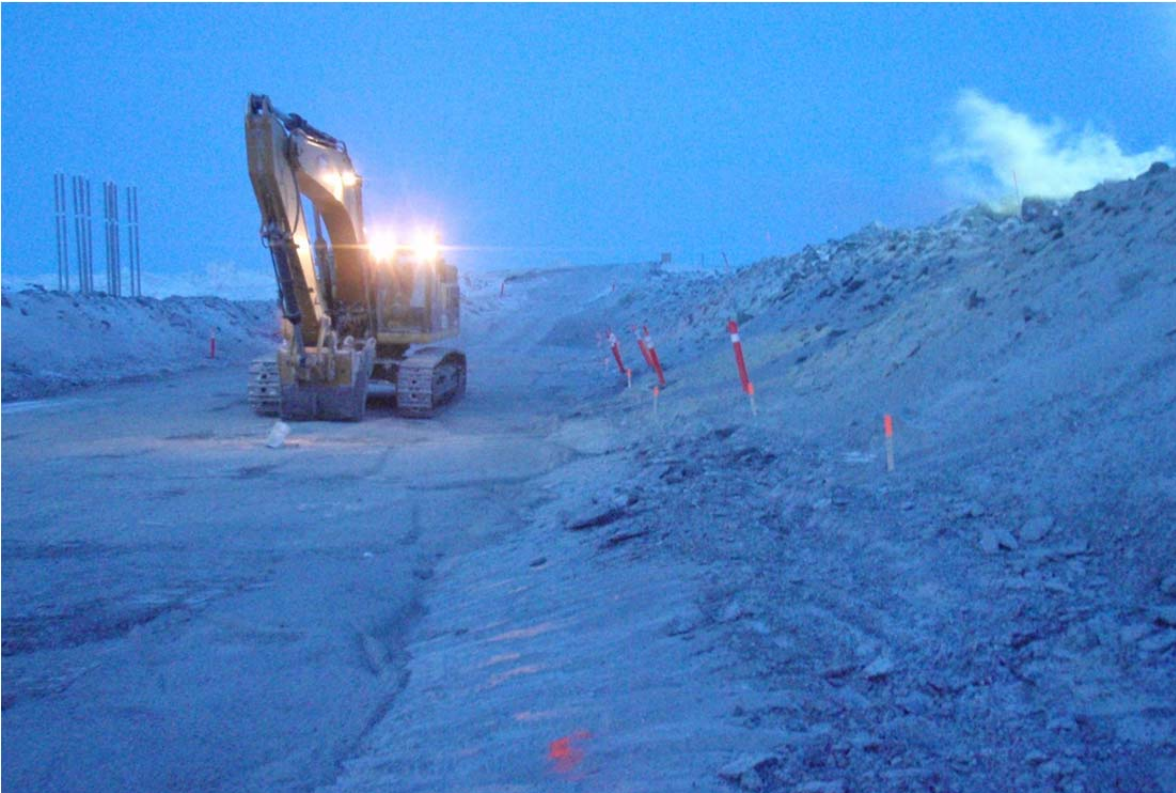
Photo 10: ~NEE view of excavator cleaning 5/8" material from the upstream fillet slope.
