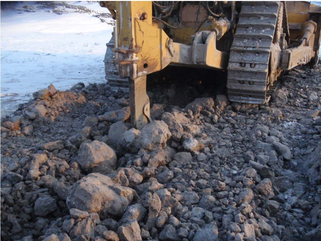
Photo 1: View of D9 ripping up frozen tundra/ permafrost along the W side of the DN Diversion Berm alignment.
