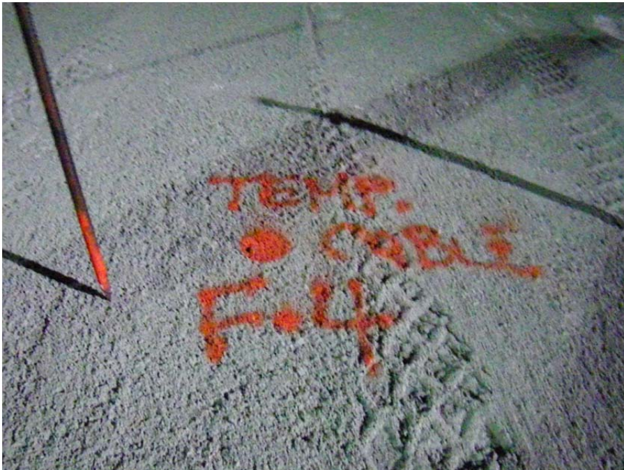
Photo 11: Paint marks indicating the height to the next horizontal thermistors cables above the current lift.
