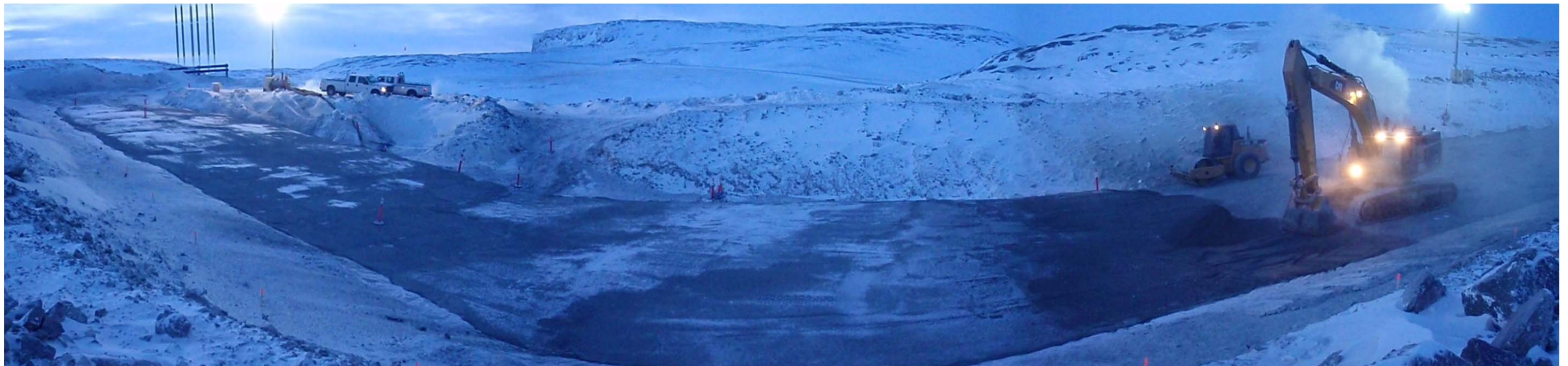
Photo 9: ~ N stitched panoramic view of FCM placement progress on dayshift, taken in the pm. Note the 345 excavator is spreading the dumped material in ~ 0.3m thick lift before it is compacted with the vibratory roller.
